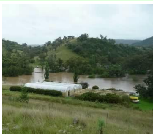
Mole Station Native Nursery at Tenterfield NSW threatened by flood waters
